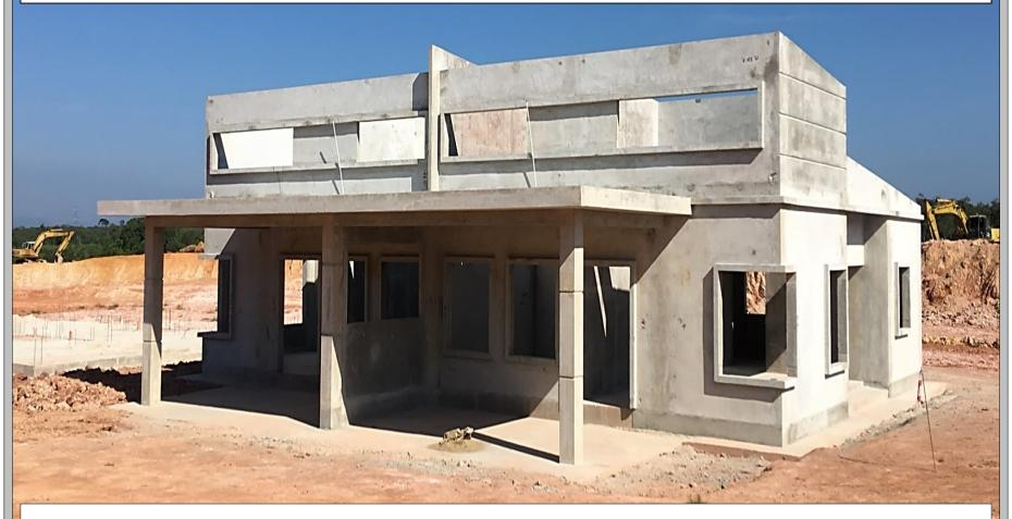
" Choose Industrialised Building System (IBS) for Economical Construction Industrialised Building System (IBS) functions as a comprehensive superstructure construction system whereby flexibility in it's customisation allows Architect's creativity to flourish."
